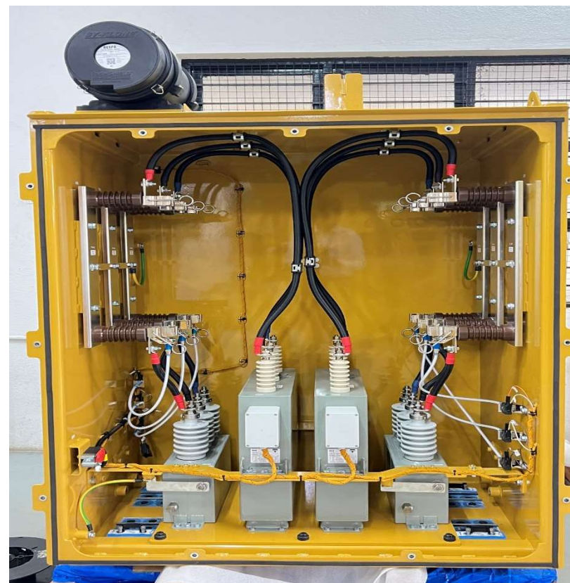
Power Factor Correction Cabinet
